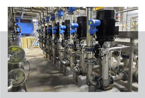
IoT and Electric Signature Analysis (ESA) provide an option to improve both these aspects radically. ESA uses pump motor current measurements to calculate various parameters, such as flow rates and motor usage. This allows for a new way to gain information on the state of pumping processes across operations.
